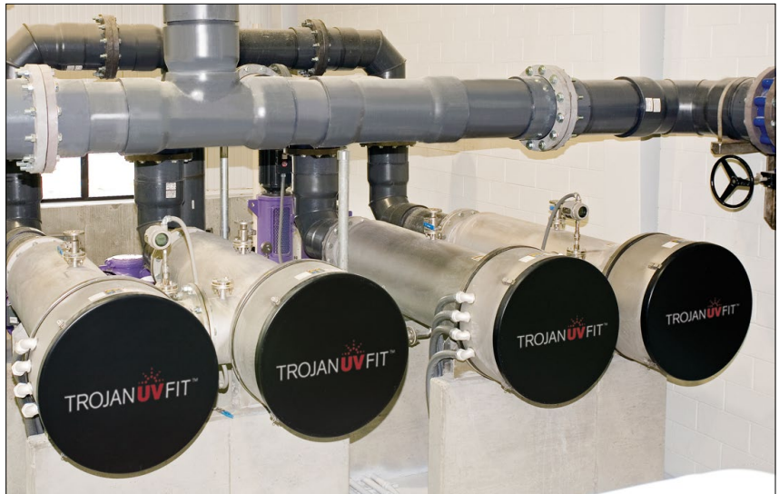
Chambers can be installed in parallel or in series for increased design and installation flexibility.
